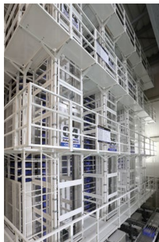
Rotary Rack H, one of the tallest in Japan
